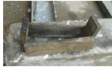
Fig .1.16 wooden mould for small size beams
