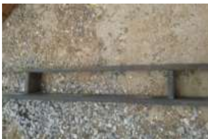
Fig. 1.14 wooden mould for large size beams
